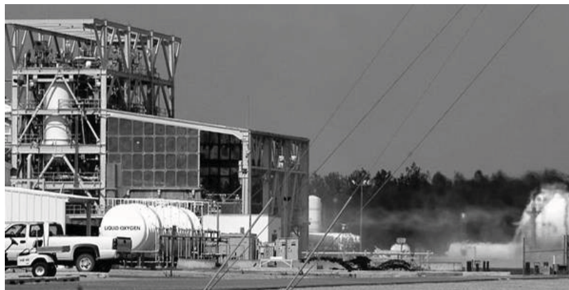
FIGURE 1. The E-1 propulsion test complex at Stennis Space Center in Mississippi consists of a component test stand, high pressure gas storage, and cryogenic storage tanks. The liquid hydrogen storage tank used for this project can be seen in the distance at the right side of the photo (distorted by rocket exhaust plume).
